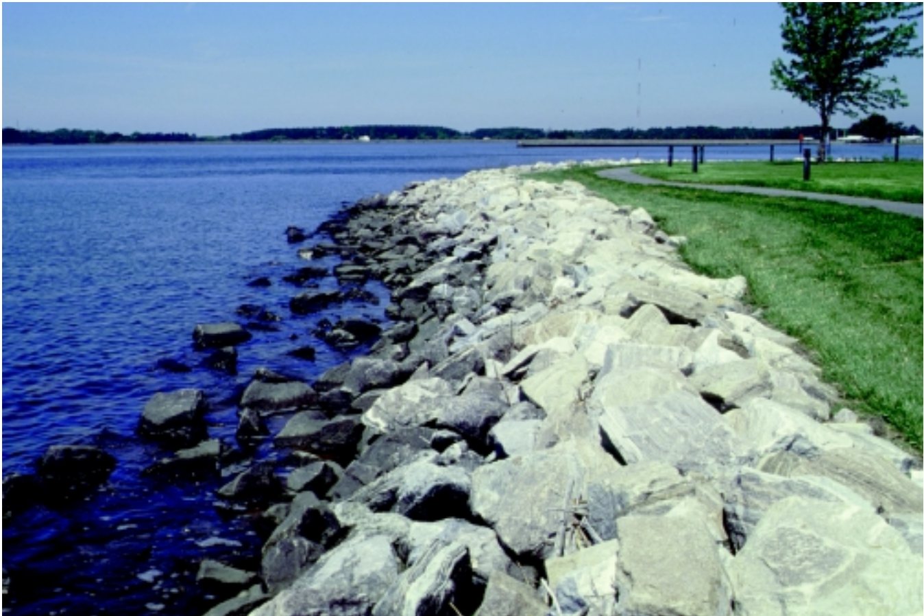
Figure 16-51 Rock riprap revetment
