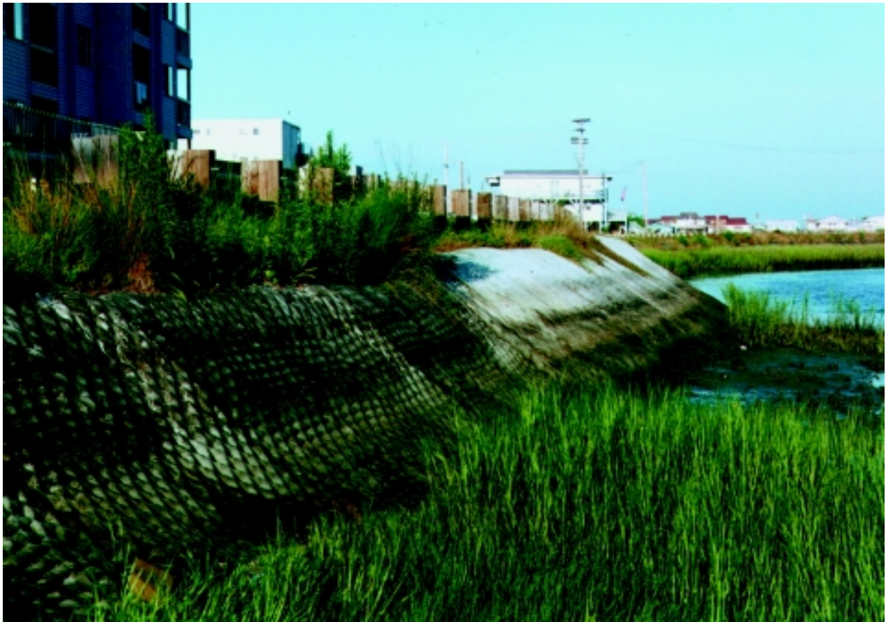
Figure 16-50 Concrete revetment (poured in place)
