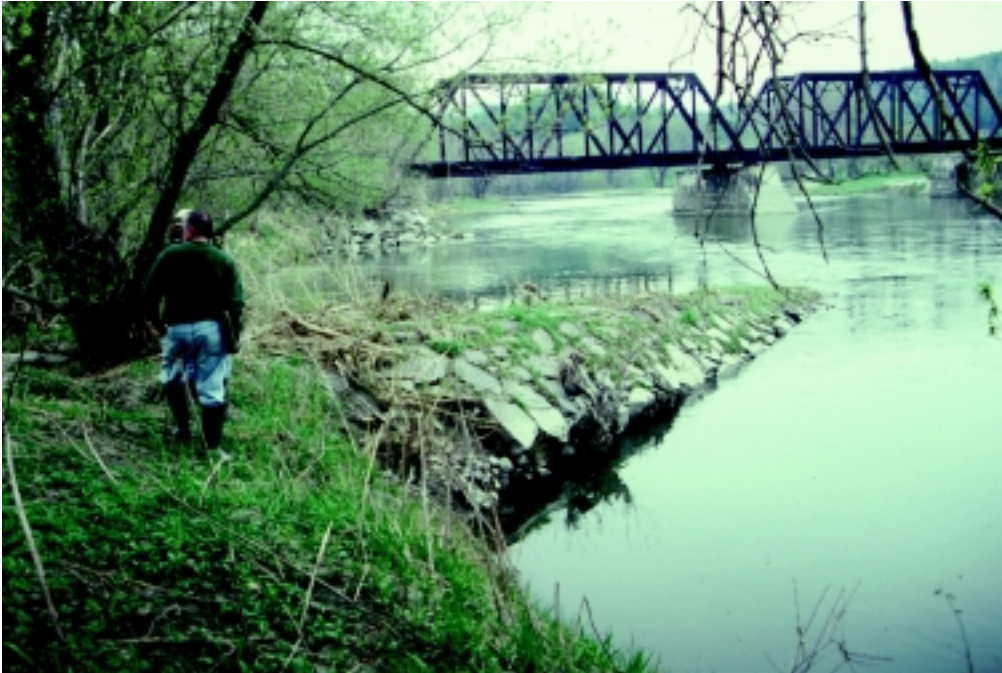
Figure 16-39a Stream jetty placed to protect railroad bridge
