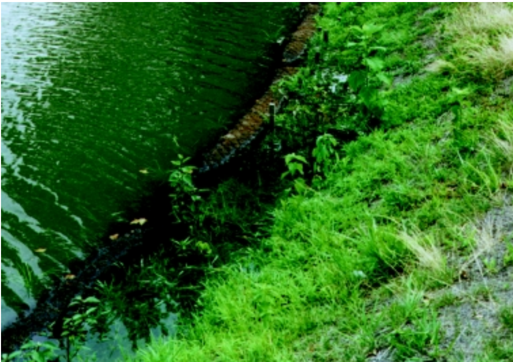
Figure 16-37b Coconut fiber roll system
