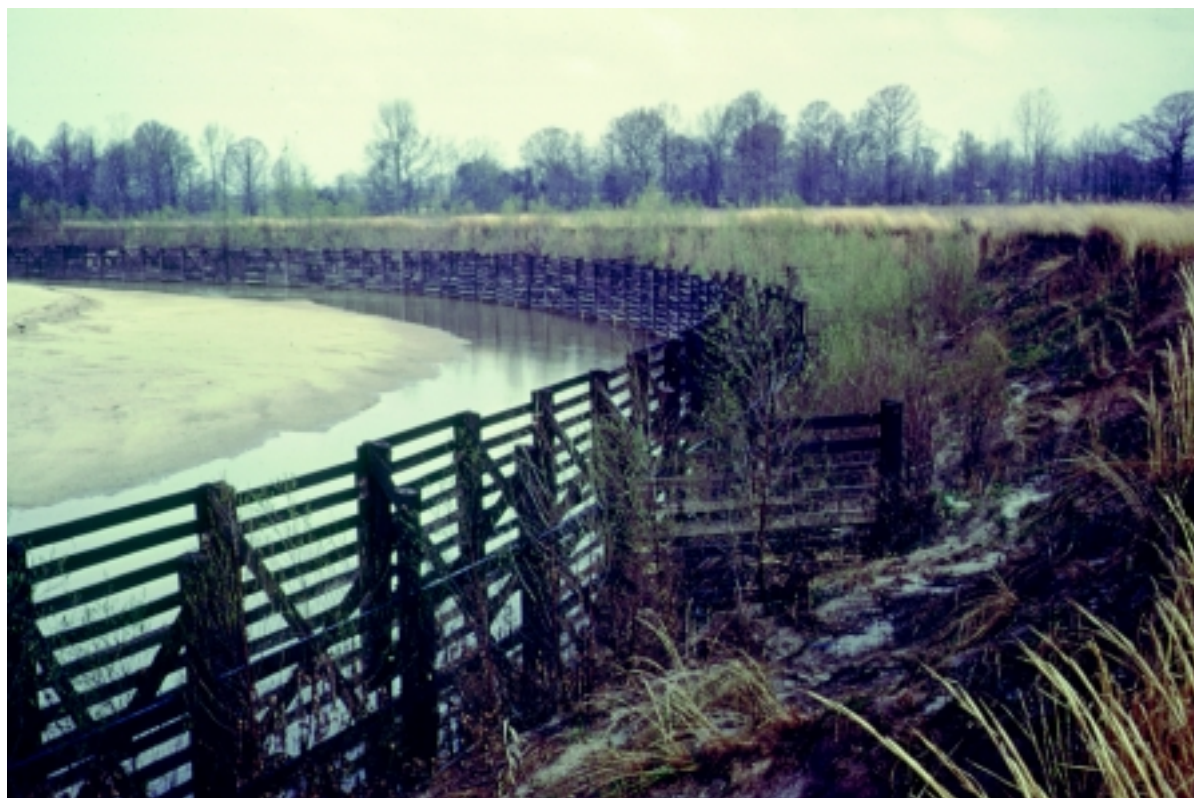
Figure 16-28 Slotted board fence system
