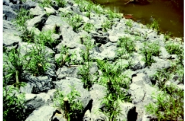
Figure 16-17b An installed joint planting system (Robbin B. Sotir & Associates photo)
