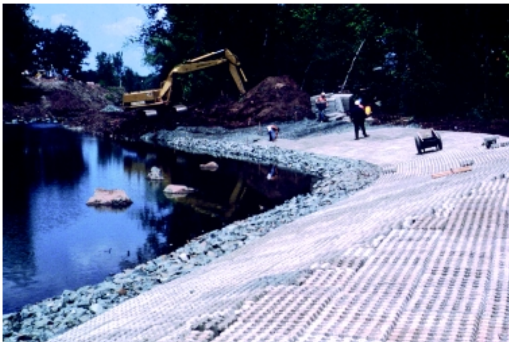
Figure 16-35a Concrete cellular block system before backfilling
