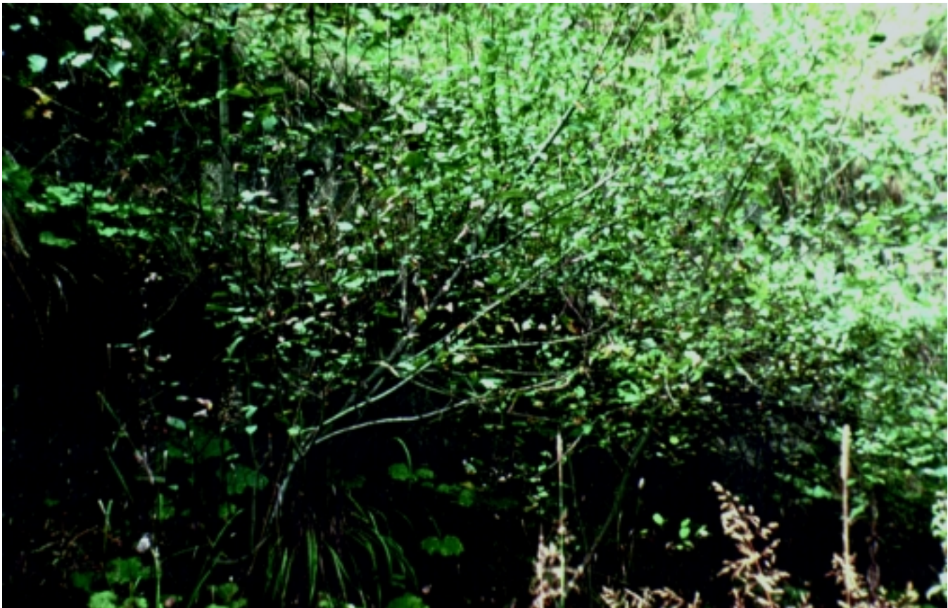
Figure 16-43 Vegetated rock gabion system (H.M. Schiechl photo)
