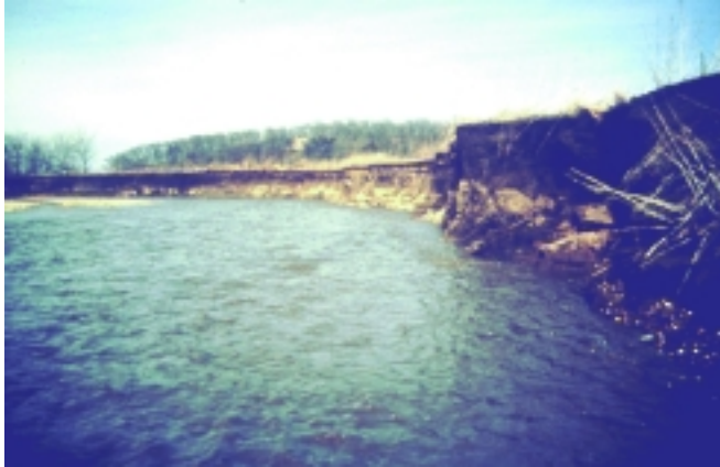
Figure 16-25a Pre-construction streambank conditions (Don Roseboom photo)
