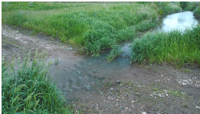
Figure 16. Example of an established hardened stream crossing.
