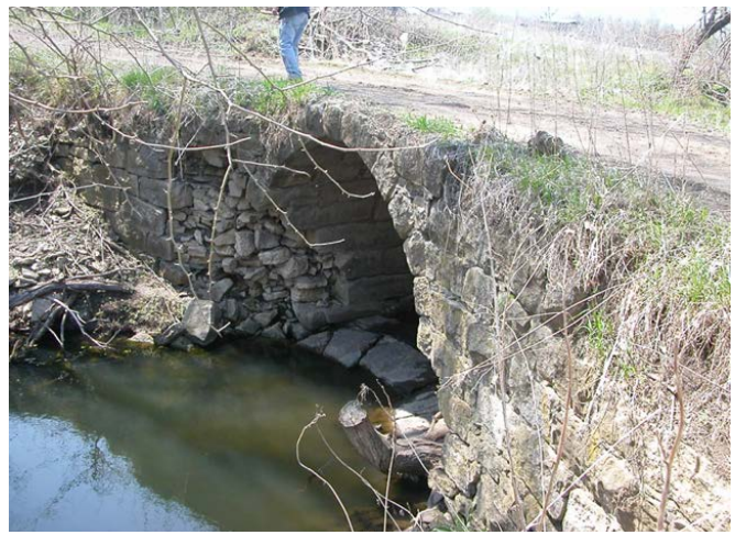
Figure 10. Many bridge and culvert problems are blamed on age, but actually are caused by undermined footings like on this stone arch culvert.
