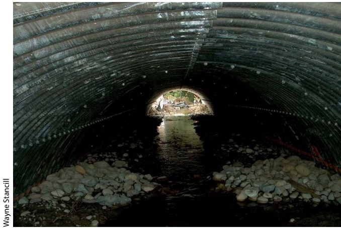
Figure 18. Rock bands reduce flow velocity in a culvert.
