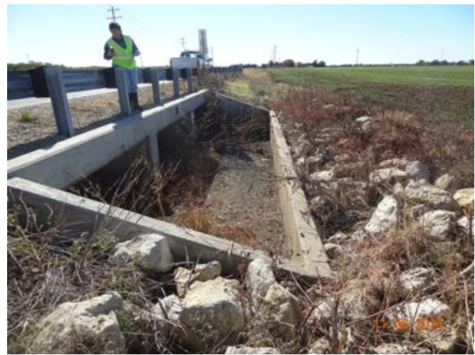
Figure 13. A typical soil saver, above, does not provide fish passage.
